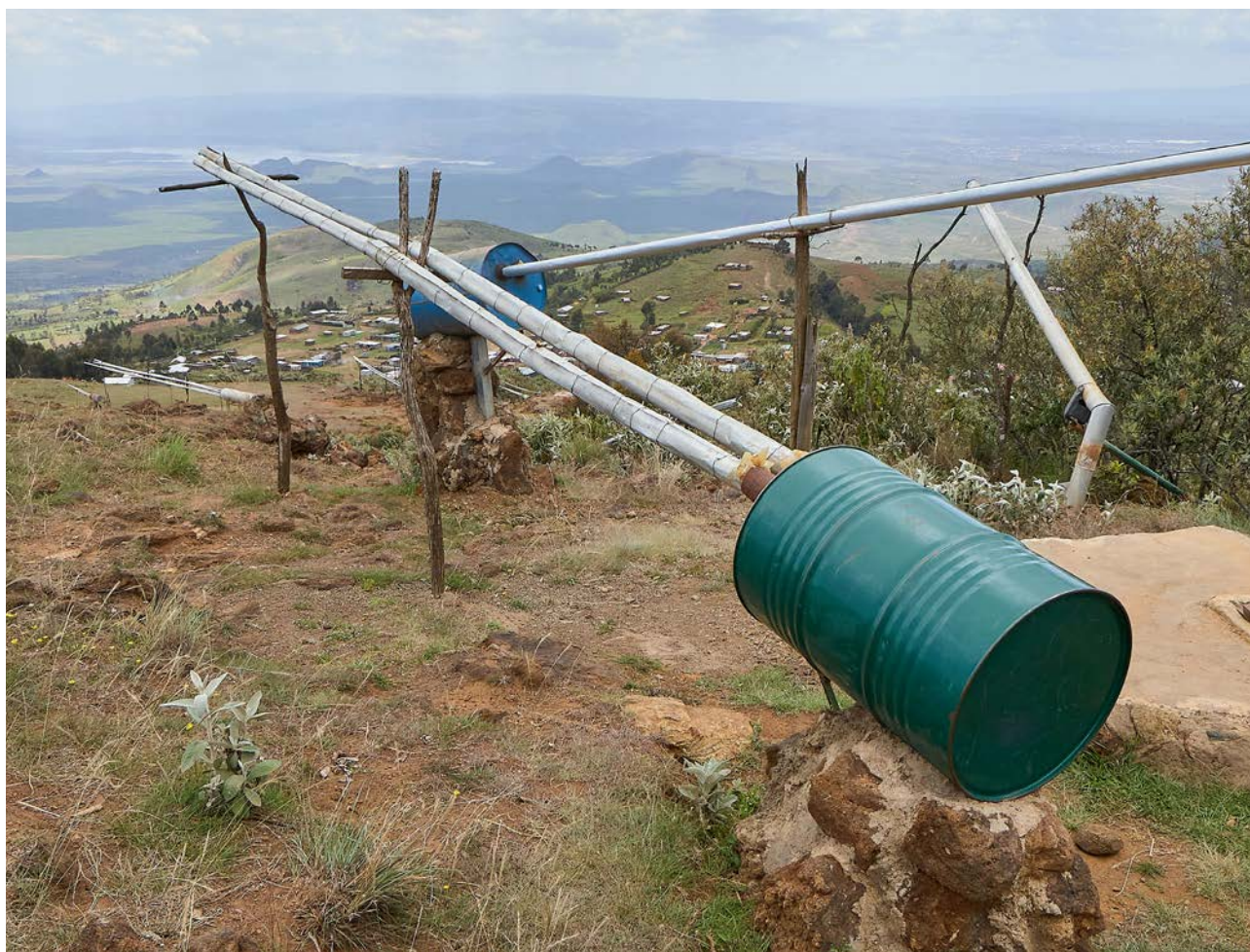
Figure 5.3. Water harvesting technology involving trapping and condensing of underground steam © KNT
